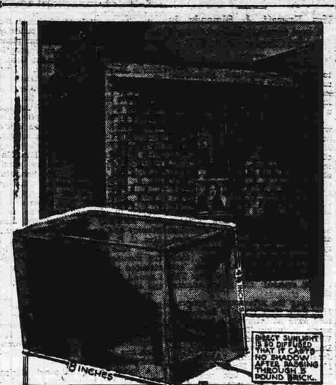
Glass houses? Yes, but they are not transparent, and they will withstand cold, wind, rain pressure and blows. Above are shown a small "Joseph's coat" factory office and one of the glass blocks from which it was built at Columbus, Ohio, for experimental purposes. Mortar joints cause curious color effects when the structure is viewed from varying angles.
